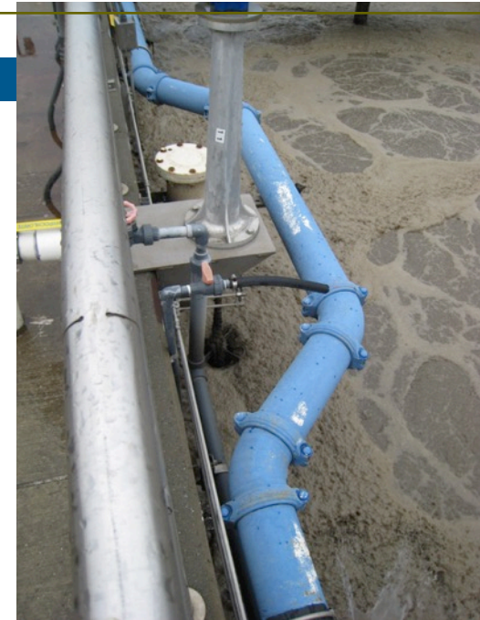
Surface Wasting – Bell Weir
