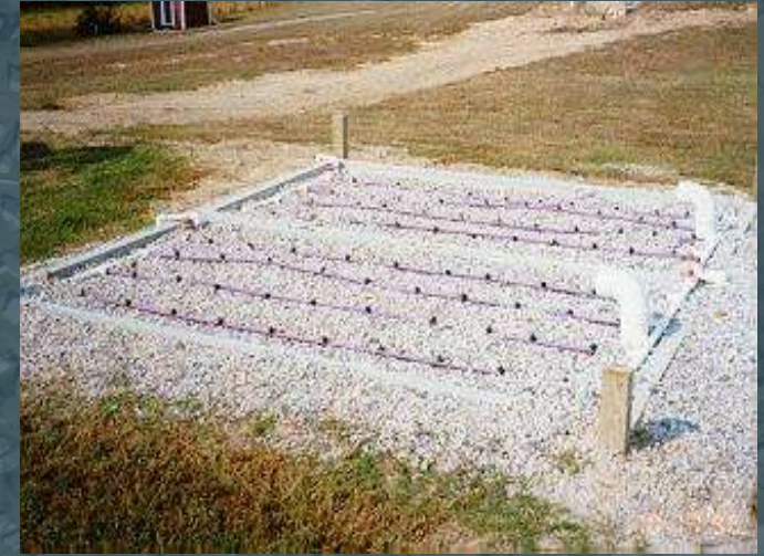
Recirculating Sand Filter
