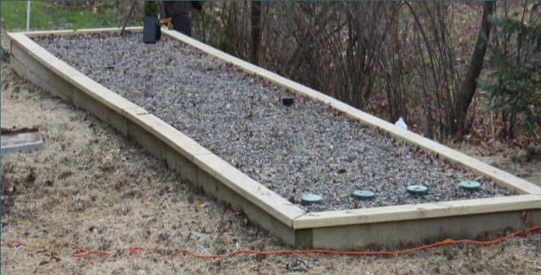
Bottomless Sand Filter - Complete
