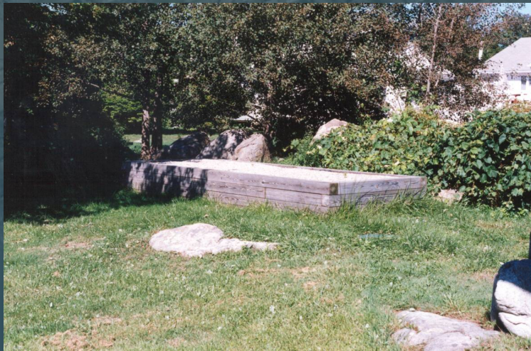
Smaller Bottomless Sand Filter
