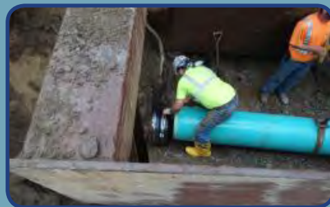
Springfield Water and Sewer Commission – Infrastructure Improvements 2014 Springfield, MA
