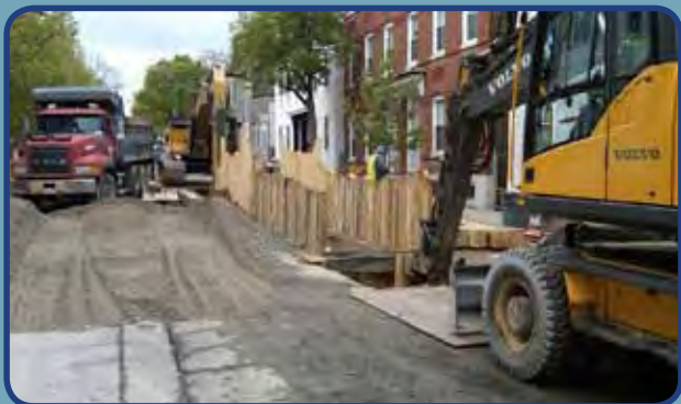
New Gravity Sewer Construction South Boston, MA
