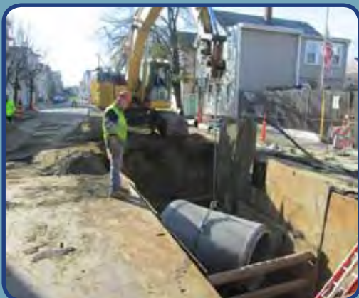
54-inch Storm Drain Installation – Reserved Channel Sewer Separation Project Boston, MA
