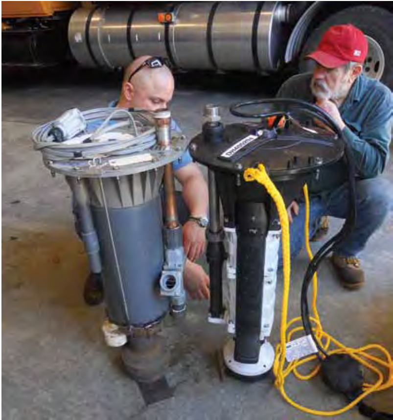
Palmer, Mass.—a newer series pump core (right) being sized up for future installation beside a first-generation series of pump
