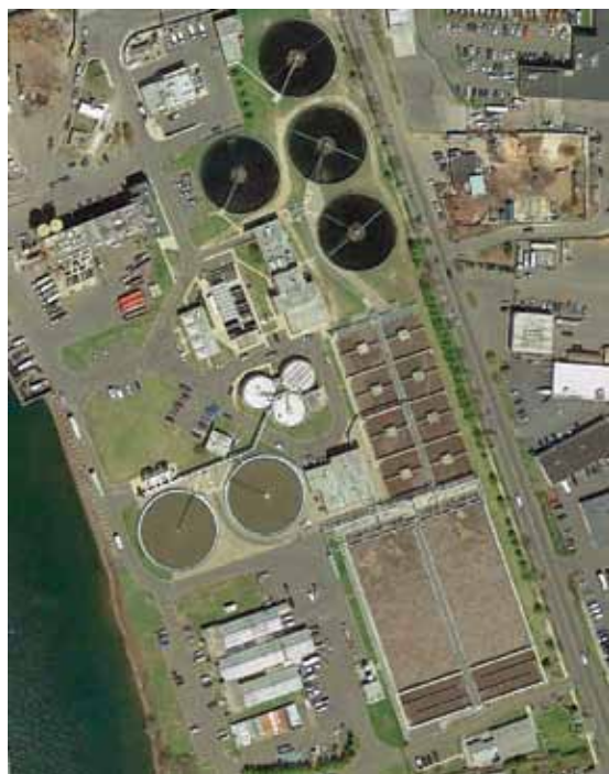
In the spring of 2014, a pilot test of a WLAN was initiated at the Stamford Connecticut Water Pollution Control Authority facility
