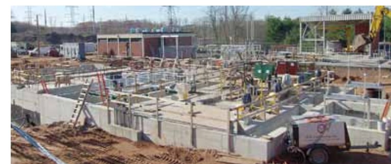
Figure 4. Tertiary treatment facility under construction
