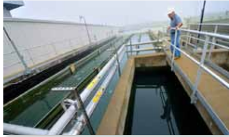
ENERGY MANAGEMENT ACHIEVEMENT AWARD Veolia Water/ Plymouth, MA WWTP
