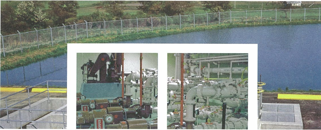
Scituate, Massachusetts: One-mgd water pollution control plant, originally designed in 1965 and upgraded in the mid 1980s to include a septage receiving facility, new aerobic digesters, and a sludge dewatering building. (1985)
