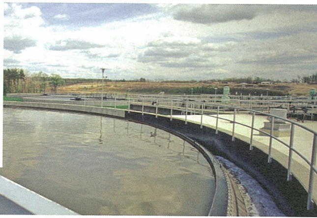
Leominster, Massachusetts: 9.3-mgd advanced wastewater treatment plant that replaced primary and secondary facilities. (1983)
