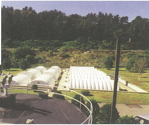
Windsor, Vermont: A 1.5 mgd Secondary Treatment with Rotating Biological Reactors (RBC). In operation since 1988..
