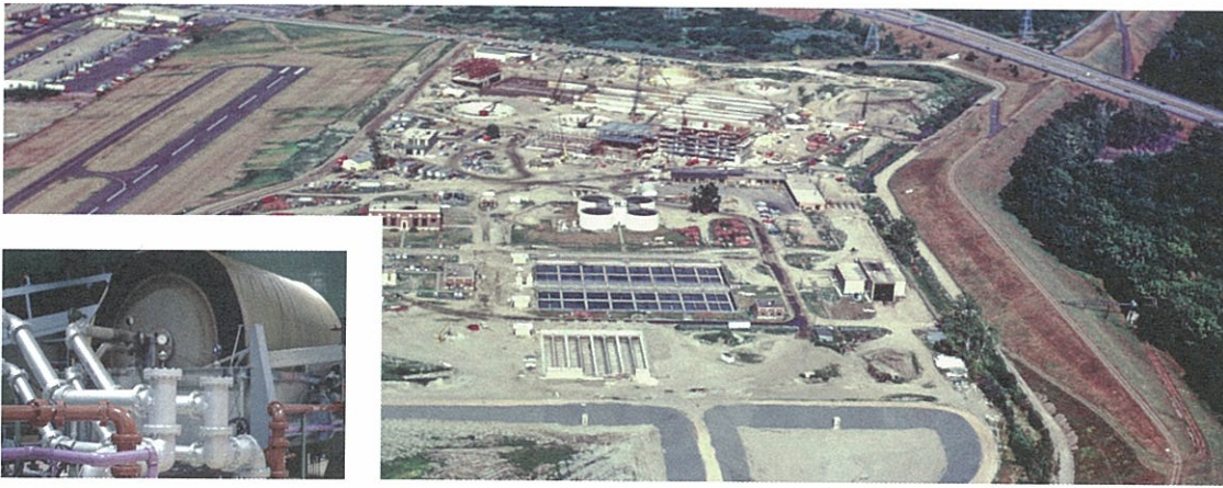
Hartford, Connecticut: The 60-mgd secondary wastewater treatment facilities in Hartford County are designed to handle an average flow of 60 mgd using the step-aeration activated sludge process. (1972)
