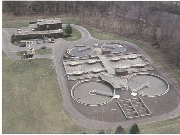
Westfield, Massachusetts: Wastewater treatment plant originally designed in the early 1970s with a capacity of 4 mgd, but has been upgraded several times since then and recently expanded to handle 6 mgd and provide nitrification and phosphorous removal during the warmer months. (1972)
